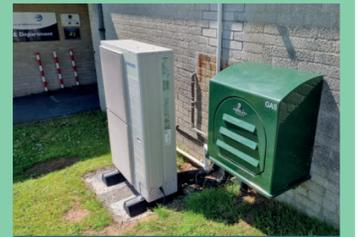
This hybrid heating system installed at the Port of Milford Haven's offices uses a heat pump powered by solar energy, but can switch to hydrogen during cold spells.
