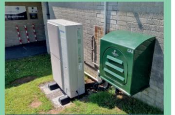
This hybrid heating system installed at the Port of Milford Haven's offices uses a heat pump powered by solar energy, but can switch to hydrogen during cold spells.
