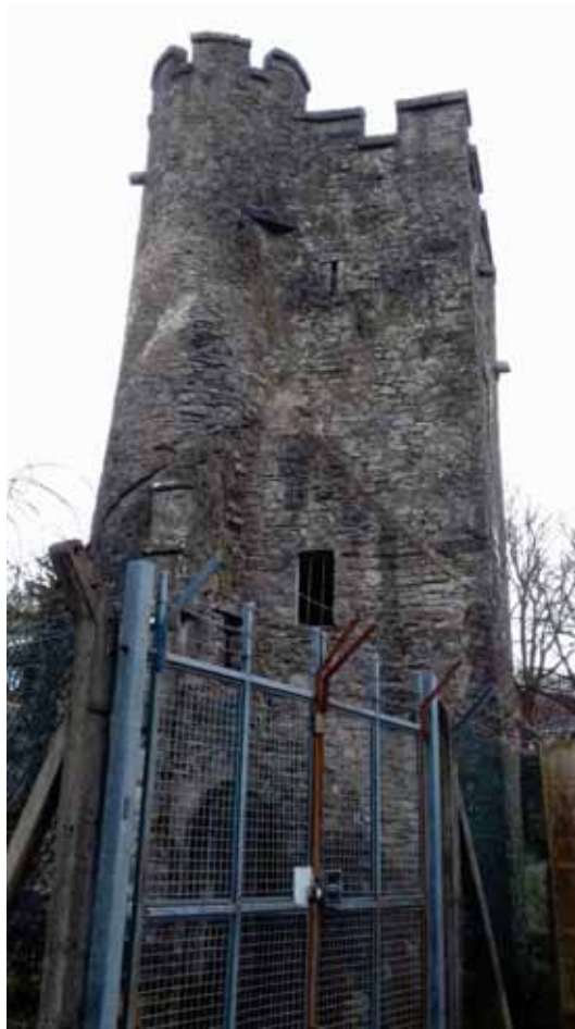
Plate 07: Disused tower, fenced off and not part of the Assessment Site.
