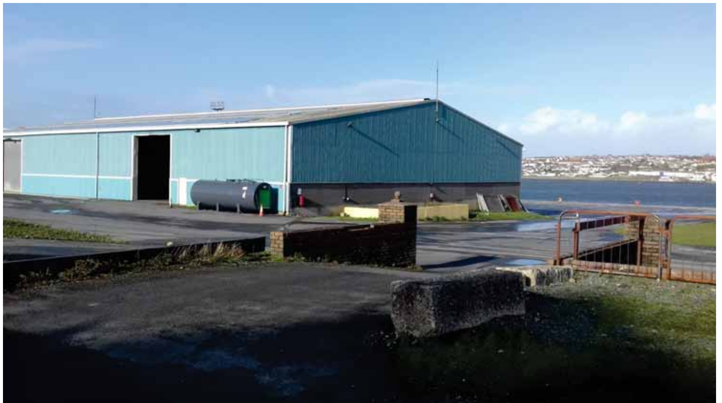
Plate 04: Facing north towards estuary. Modern diesel tank on warehouse corner. Former tank bund (yellow) adjacent.
