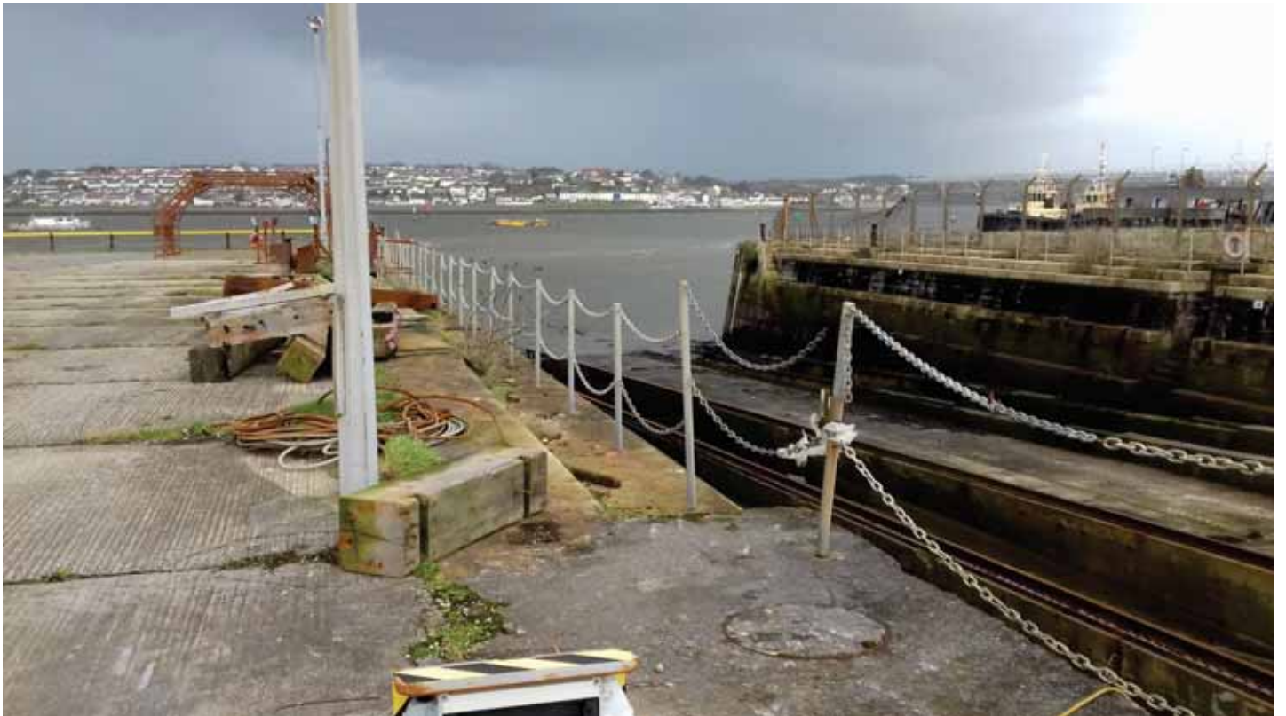
Plate 16: Facing north towards the estuary. Showing Slipway 2.
