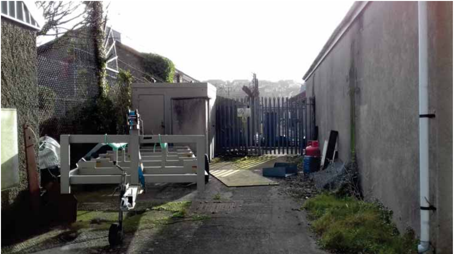
Plate 22: Electrical sub-station present between Slipway 2 and 'triangle' area of land not owned by MHPA.
