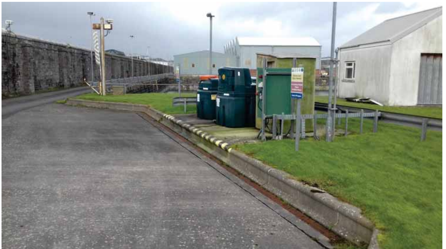
Plate 14: Fuelling point in southwest corner. Facing north.
