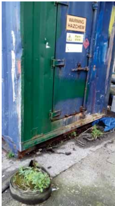
Plate 17: Gas supply control valve, south of Slipway 1. Facing northwest.
