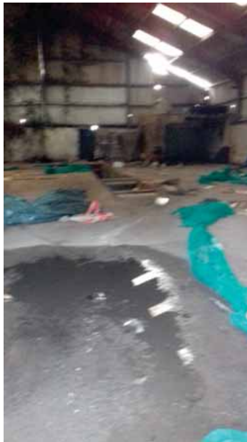
Plate 10: Possible inspection pit in floor of disused warehouse at Milforge Site.
