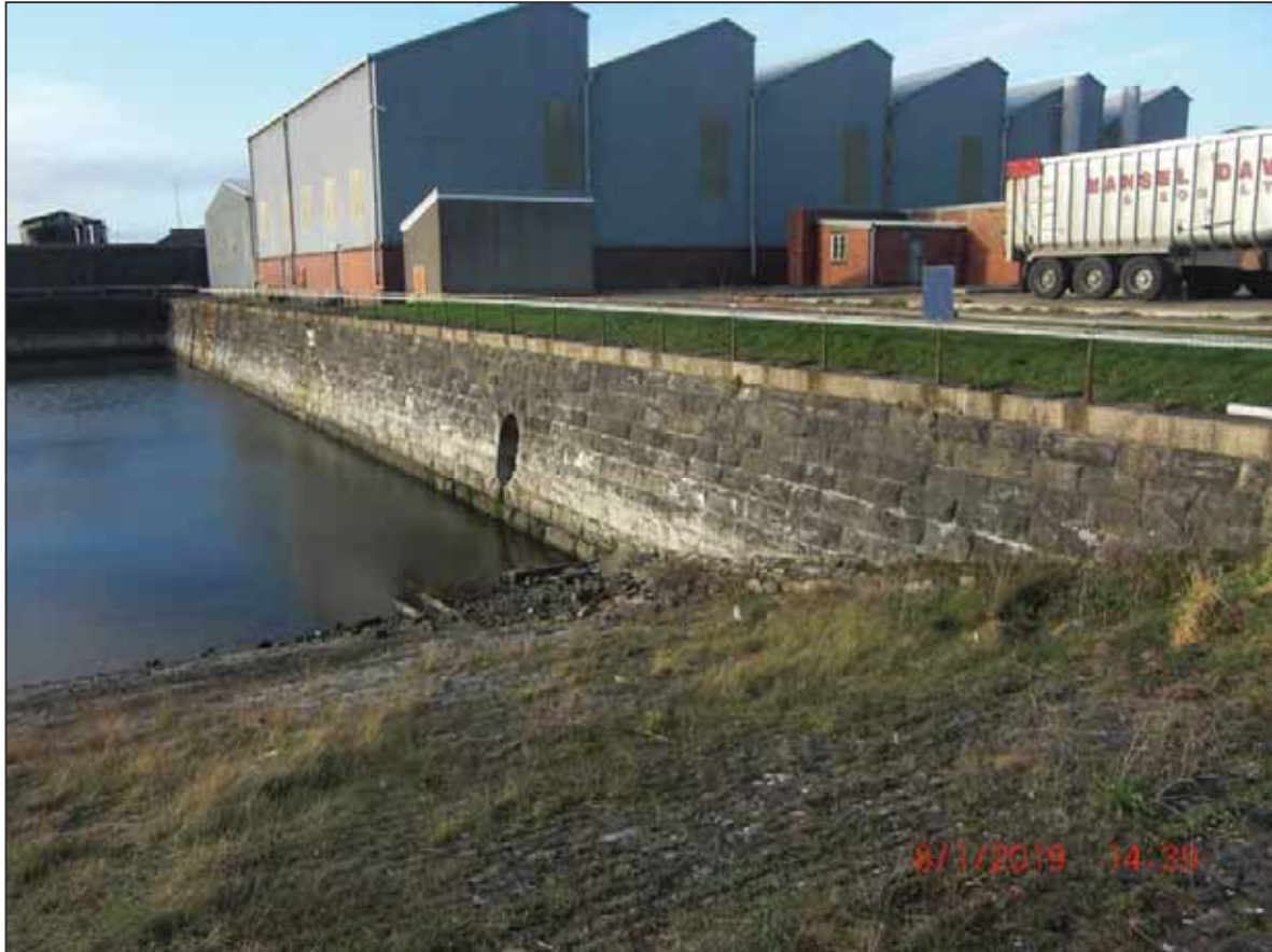
The northern wall of the timber pickling pond with Unit 29 behind.
