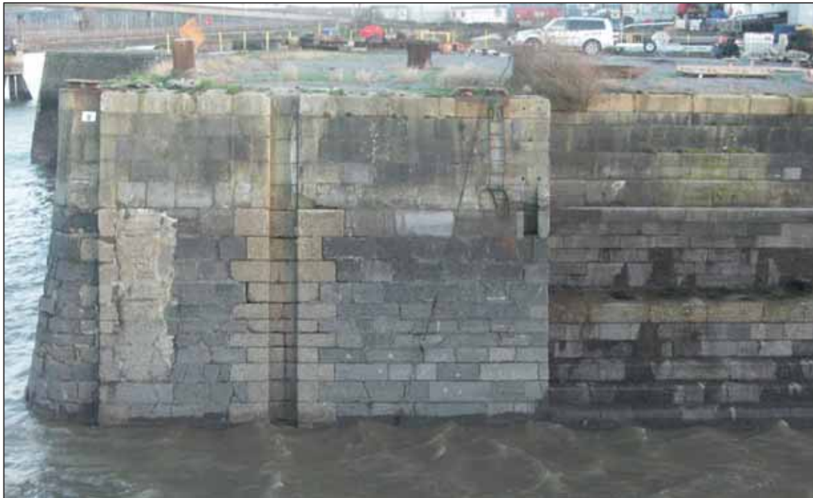
The entrance to the graving dock which will be maintained under the preferred option
