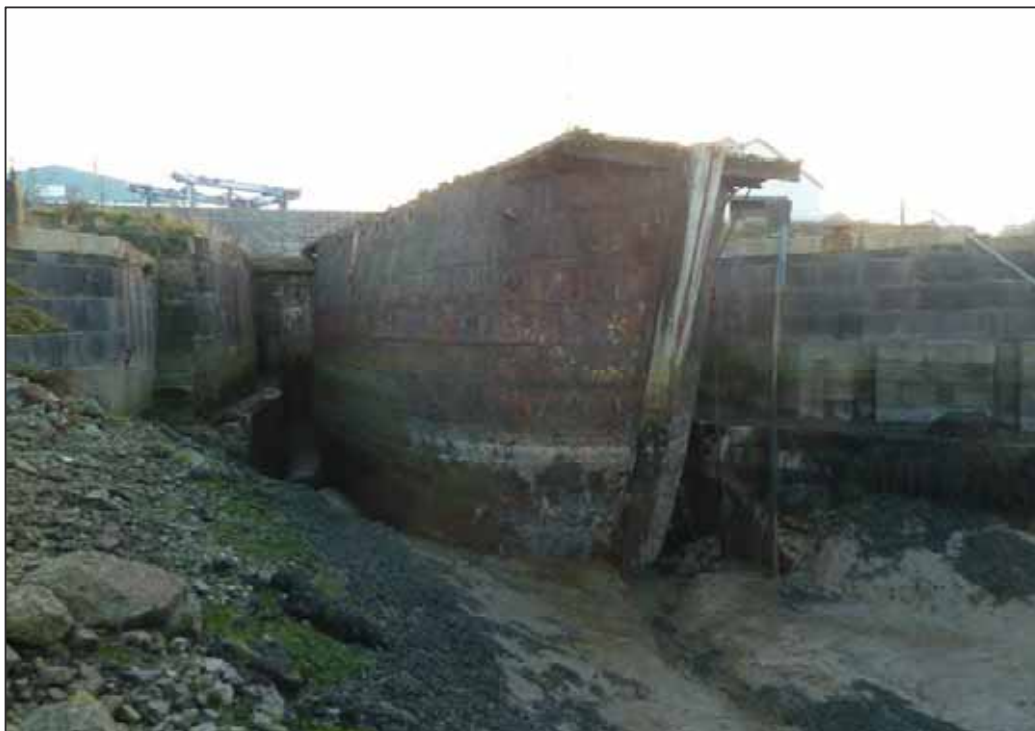
The existing caisson gate
