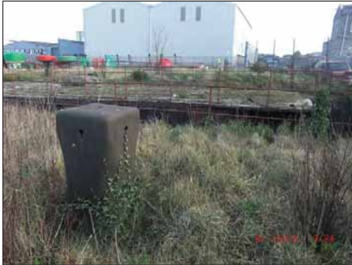
Existing iron bollard on the east dock wall
