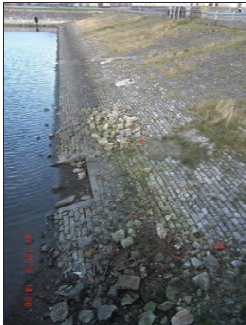
Sloping stone revetment to the east side of the pond
