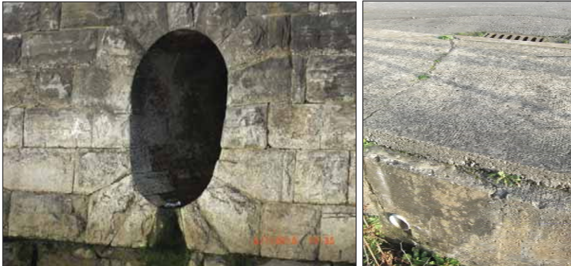
Existing culvert outlet on the north wall and a road gully and outlet on the east wall
