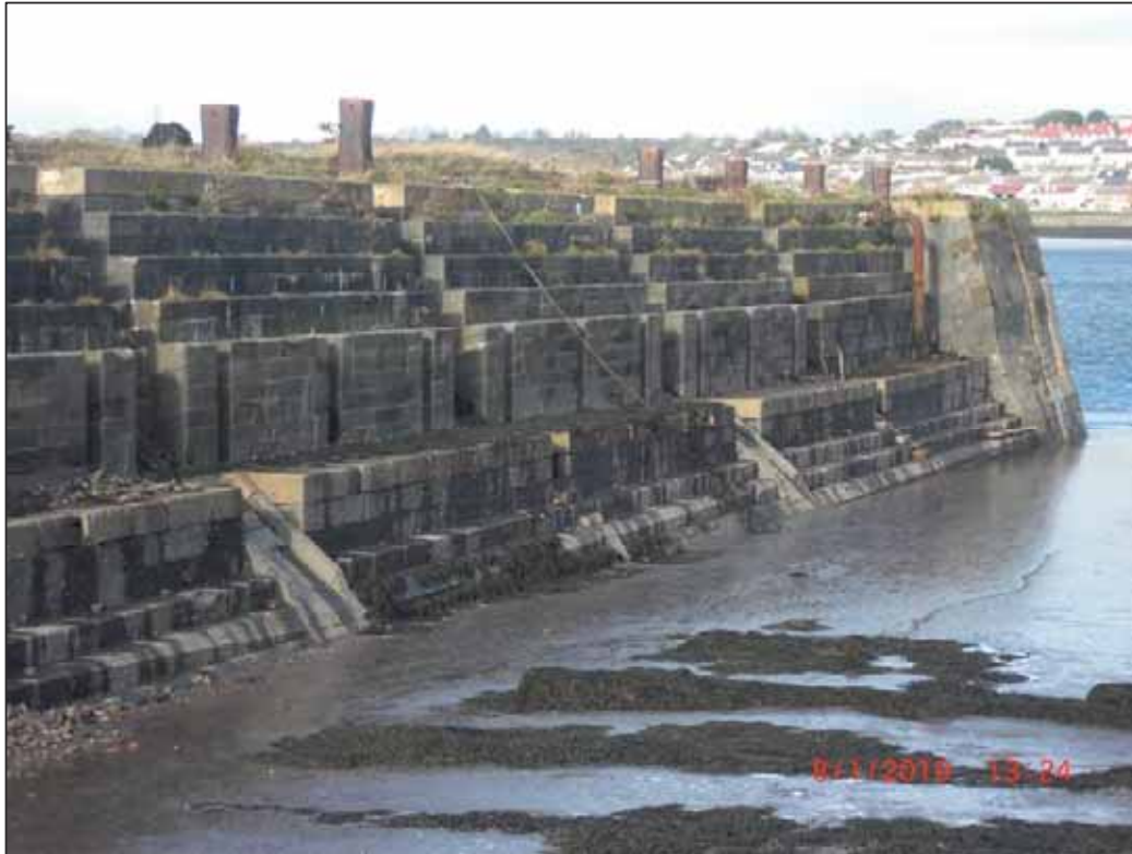
West side of the graving dock showing the limestone ashlar altars
