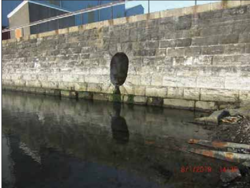
View of the north wall including the culvert outlet
