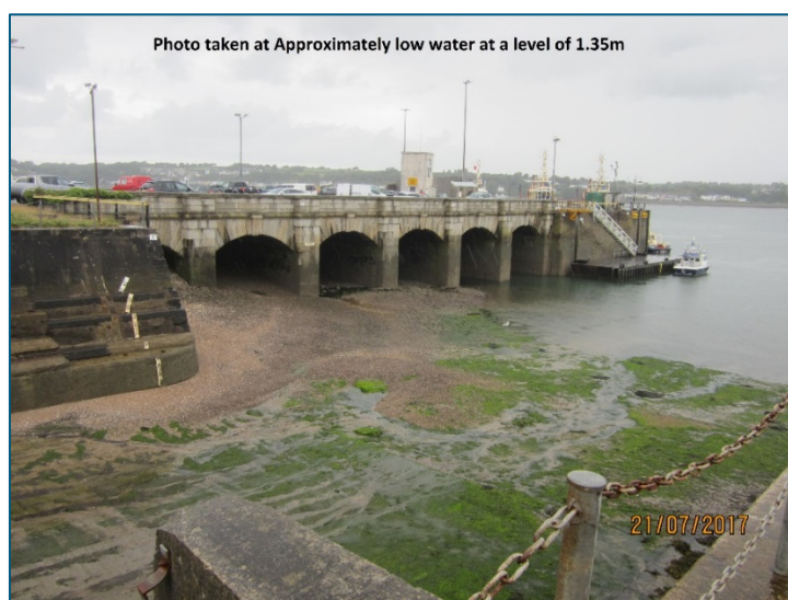
Figure 2 – Lower Section of Slipway No 1 showing Carr Jetty beyond
