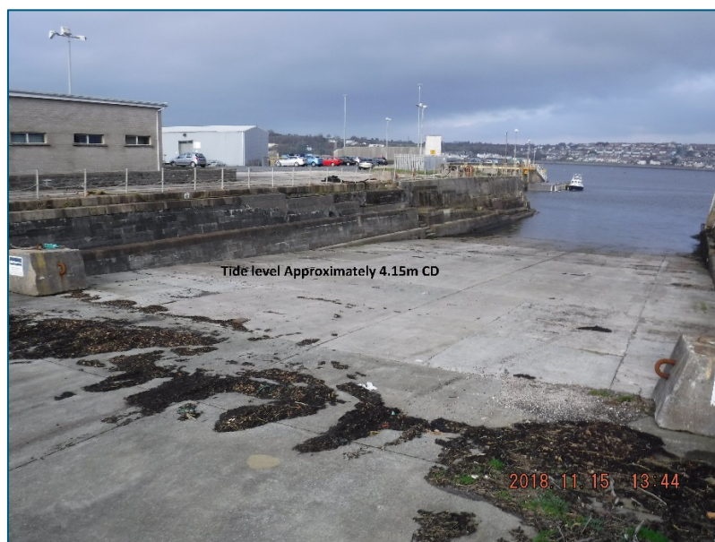
Figure 1 - Upper Section of Slipway No 1
