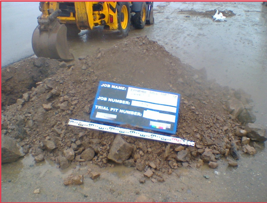
Above:- TP12A spoil
