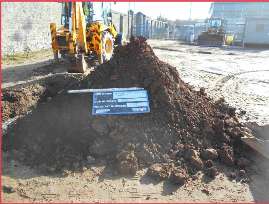
Above:- TP13 spoil
