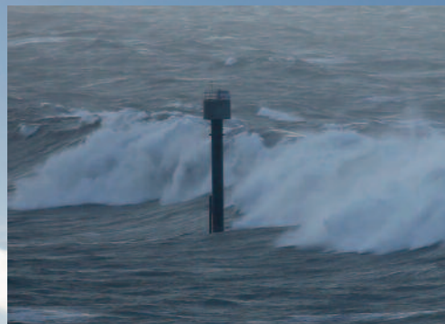
↑ All equipment takes a beating in stormy weather. The Mid Channel Mark gets pummelled by waves as high as 16m.
