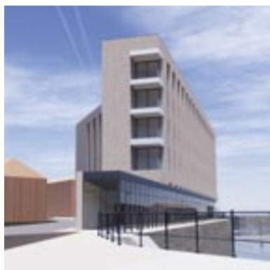
Here to stay 100 bedroom hotel gets the go ahead at Milford Waterfront
