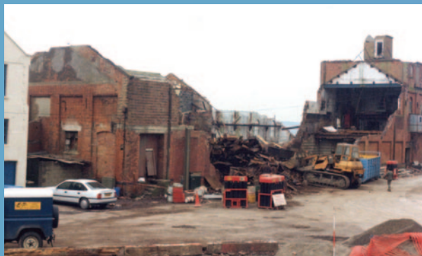
↑ The old Ice Factory, its brickwork badly damaged by constant freezing temperatures, had to be demolished
